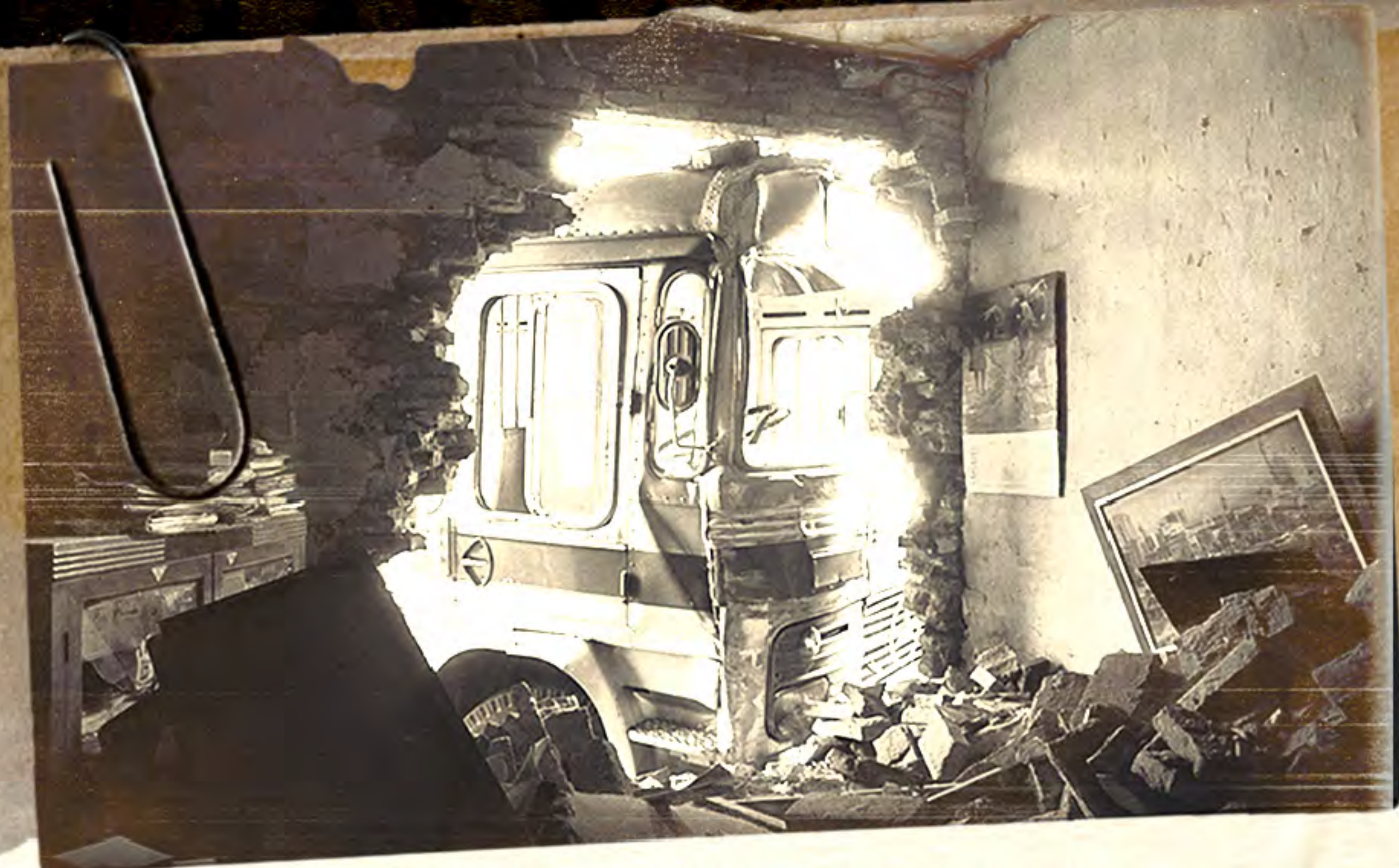
THE DESTROYED BUILDING 被巴士撞毁的建筑物
